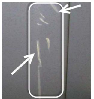
Paint is scraped and gouged. This presents an unacceptable appearance.
