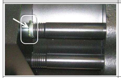
Coverage of paint on adjacent materials has gaps. This presents an unacceptable appearance. Also, primer and substrate are showing which can lead to corrosion.
